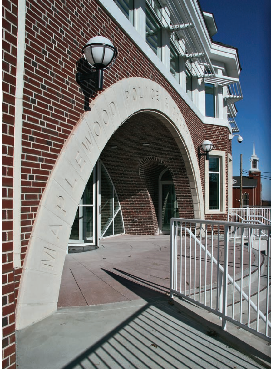
A grand masonry vault marks the building's main entrance. Exits are located under cross-vaults, one of which is visible here.
